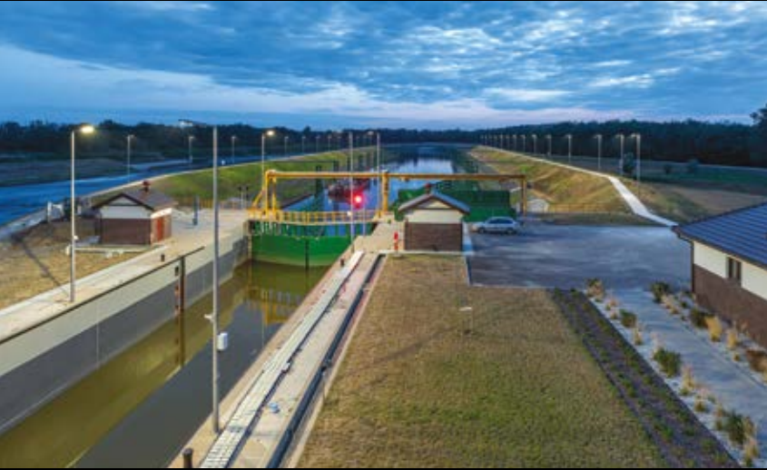
Water barrage Malczyce, Poland
