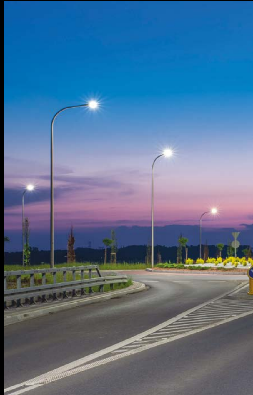
Nothern bypass of Jaworzno Jaworzno, Poland
